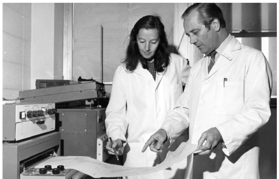
JENNY AND RICHIE NAIRN REVIEW A SPECTROPHOTOMETER TRACE ASSESSING FLUORESCENCE MICROSCOPE FILTER PERFORMANCE. C1982
