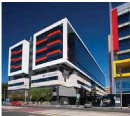
Fig 1: The Burnet ImmunoMonitoring Facility in Melbourne.
